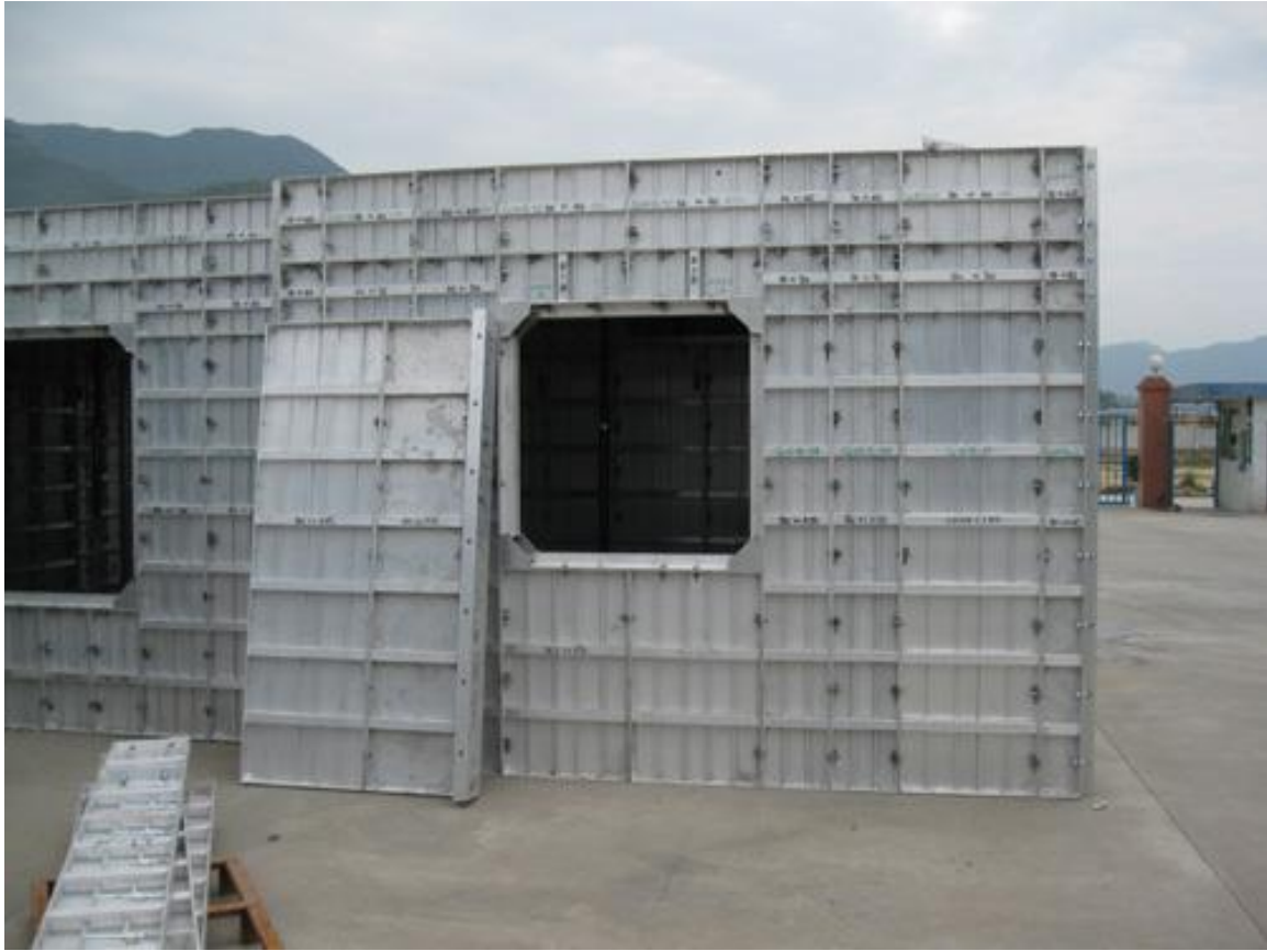
Aluminium form work system
